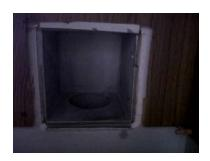
Depending on the build-up, a majority of the lint will lift off without too much effort. The vent screening should then be vacuumed to remove as much of the remaining lint as possible. Depending on the condition of the lint screen, you might wish to wash the screen with clean water.
