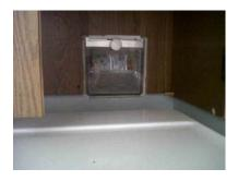
To remove the lint trap lift up on the knob so the base clears the bottom track. Once clear, lower the vent over the bottom rail and the unit will lift out. Depending on the degree of lint build-up, this may be a little messy.
